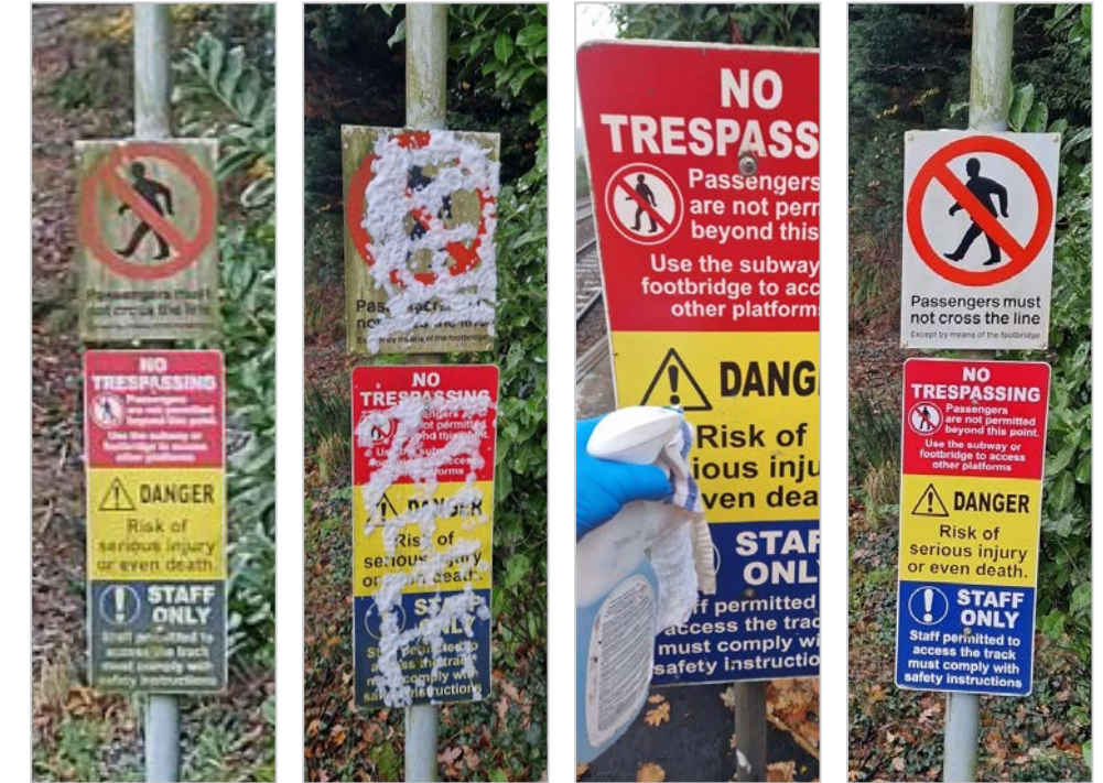
High level cleaning at Helmshore station, Greater Anglia
